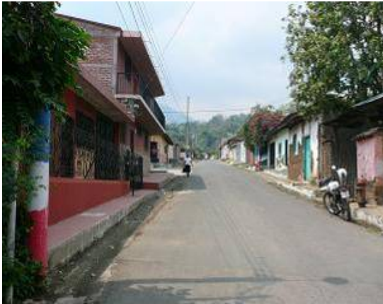
A road newly equipped with sewer pipes in Chinameca
