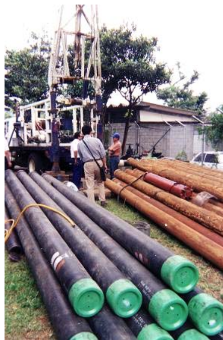
Replacement work of a motor and a pump
