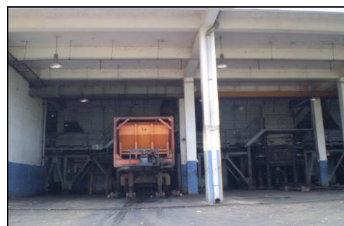
Sunter relay station
