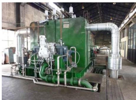
Figure 6: Gas Compressor after the Repair
