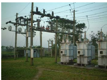
Figure 1 Substation of PBS Headquarters
