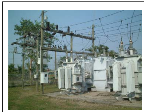
Substation of Khulna PBS Headquarters
