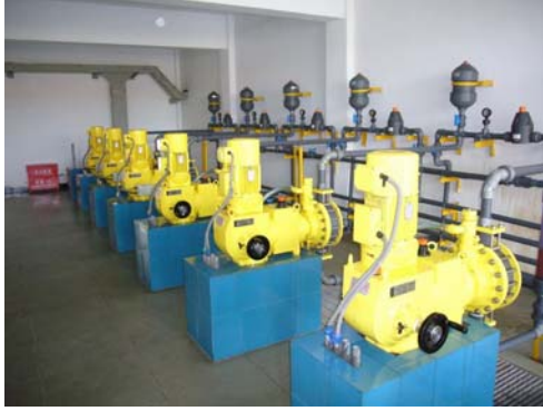
Chlorine dosage facility at Fengshouba Plant
