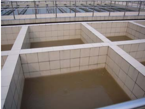
Settling tank of Fengshouba Plant
