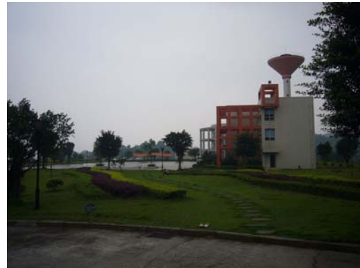
Fengshouba Water Plant
