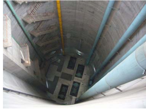
Receiving well of Fengshouba Plant
