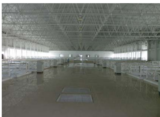
Water Purification Plant
