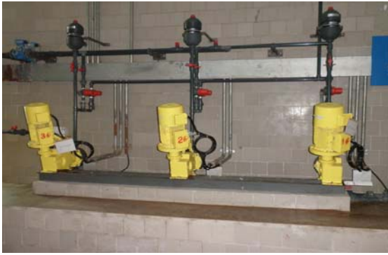
Chlorine dosage facility
