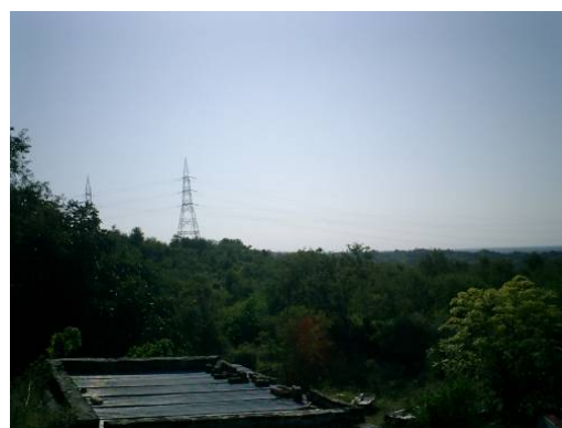
Transmission line built in the forest area
