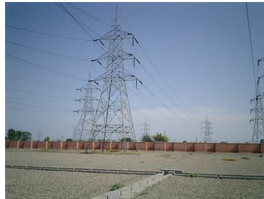
Jalandhar-Hamirpur Transmission Line constructed by this project
