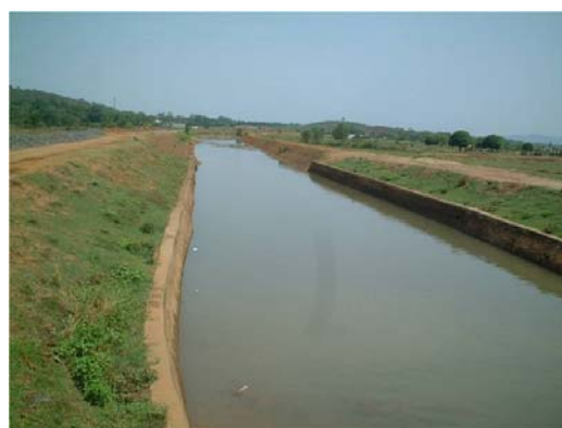
Main Canal developed by the Project
