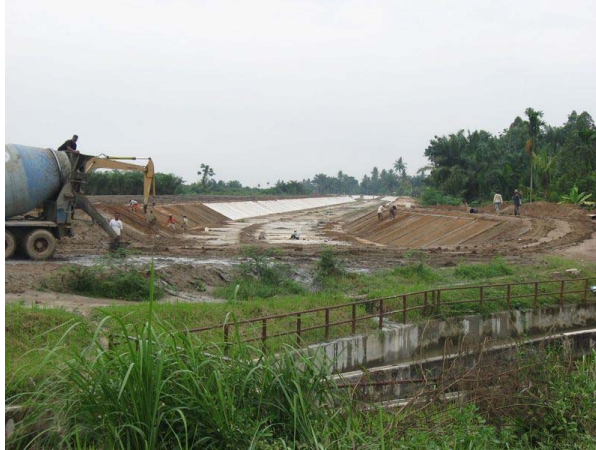
Link Canals under Construction in Ular
