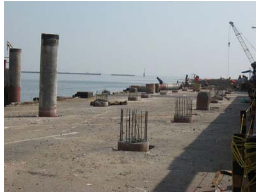
Pile foundation construction site
