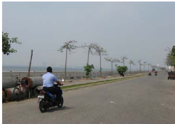
Completed east revetment water walls (July 2009)
