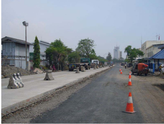
Improvement of port inner roads
