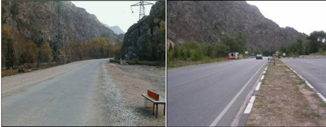
The road before construction rehabilitation (Photo by project consultant)
