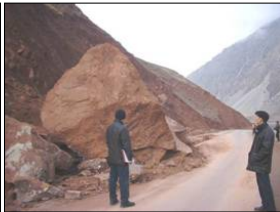
Rock fall during construction (Photo by project consultant)
