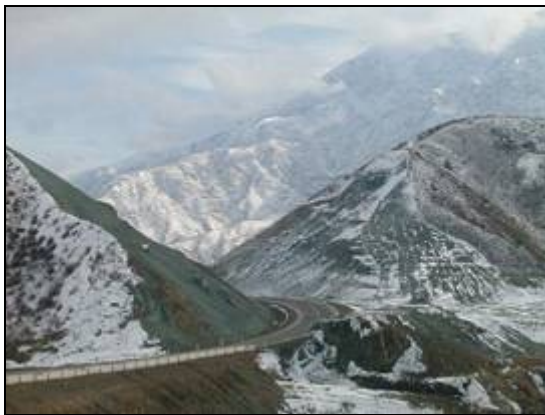
Kok-Bel pass in winter (Photo by project consultant)
