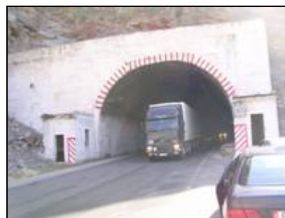
Tunnel constructed at 415km point from Bishkek
