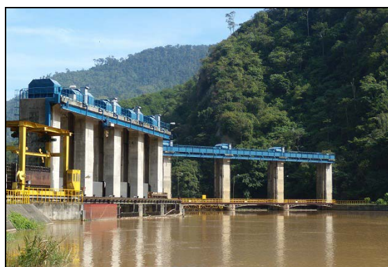
Water intake gate of the Tenom Pangi Hydropower Station
