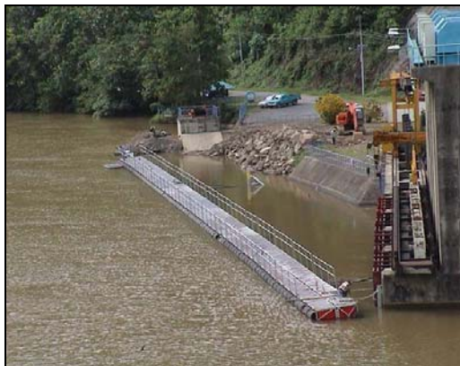
Photo 2: Water intake gate after the ex-post evaluation
