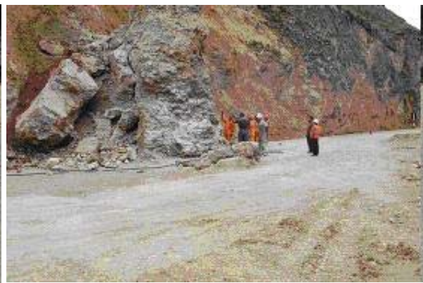
Removal of Fallen Boulder (Jauja-Tarma Highway)
