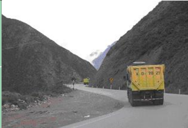
La Oroya-Huancayo Highway
