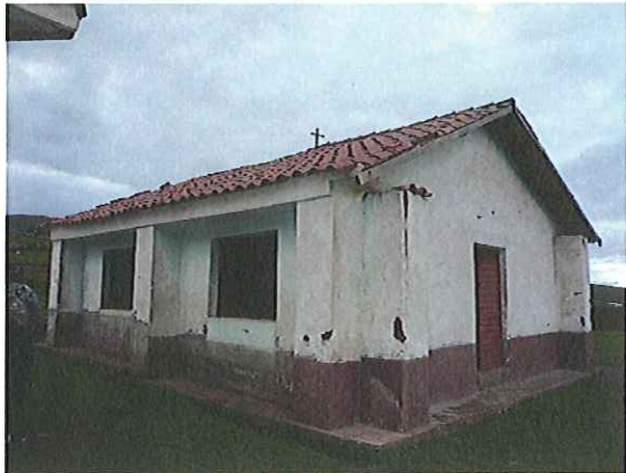
Small Warehouse (Cusco)
