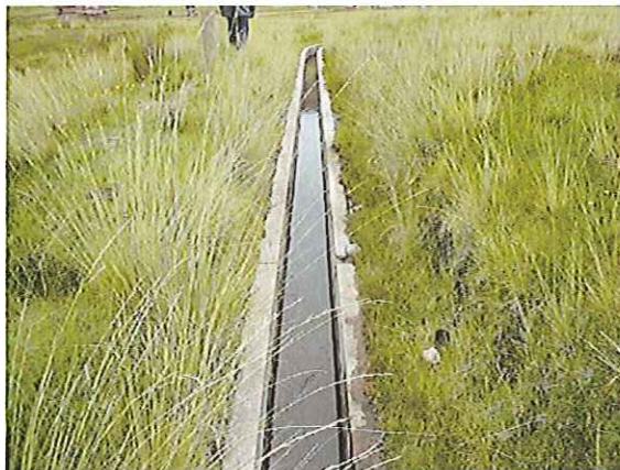
Improved Irrigation Channel (Cusco)
