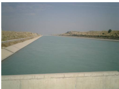
Intake water channel
