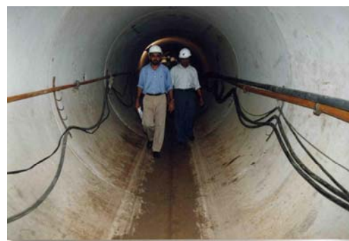
Underground drainage pipe at Unity Place
