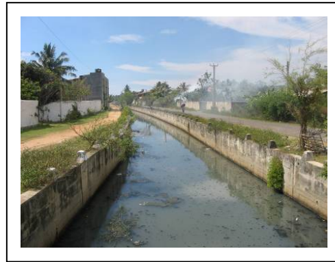
An improved drainage in Kaudana area
