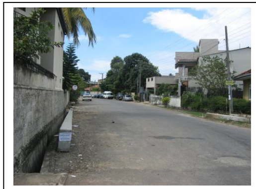
Inundation damages were reduced drastically after an underground drainage was constructed by the project (De Soysa road)
