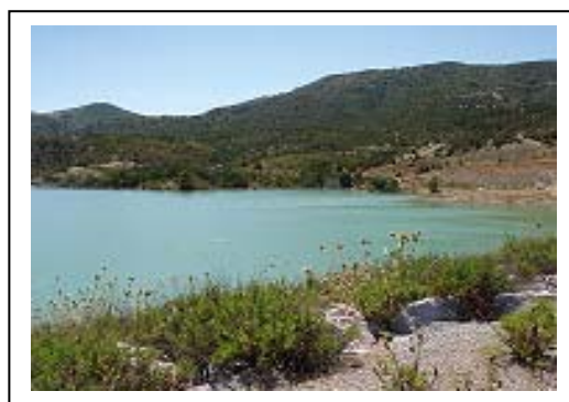
Kseub Hill Dam
