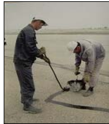
Photo 1 : Repairs with bitumen
