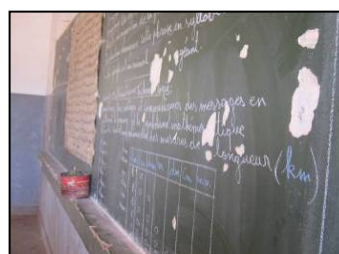
Photo 8 Blackboard with Damage Surface
