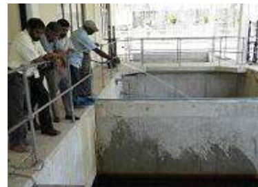
Malimboda Filtration Pond
