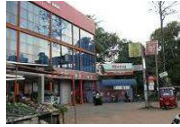
Kekanadura area, Devinuwara Division
