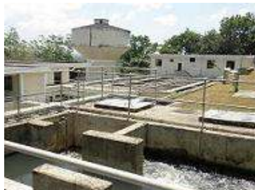
Malimboda Distribution Chamber
