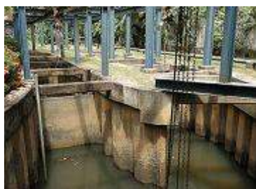
Kadduwa Intake Channel (Left: Existing, Right: New)
