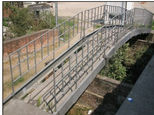
Photo 4: Underground Transmission Line Cable (at river-crossing point)
