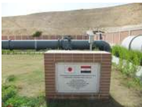
Entrance of El Rameya Water Distribution Station
