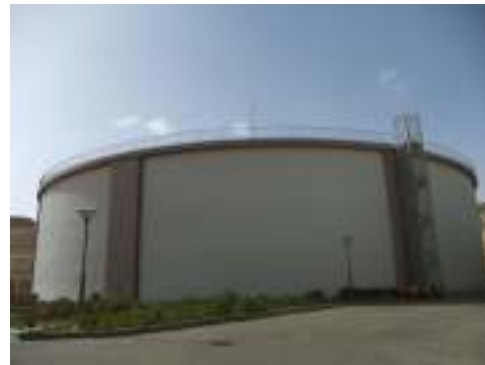
El Rameya Water Distribution Station
