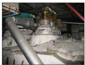
Photo 2: Inside of Steam Turbine of Unit 3 (Steam Valve)
