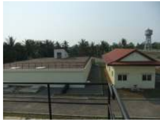
Reservoir(left),Pomp Station (right), Elevated Water Tank(back right)
