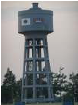
Elevated Water Tank
