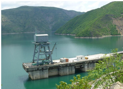
Figure 6: Intake (Reservoir Dam at Fierza Hydropower Station)
