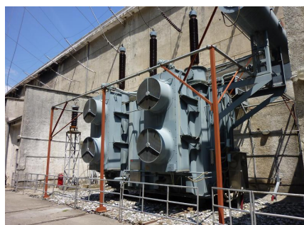
Figure 9: Generator Step-up Transformer 23 (Adjacent to Power Generation Building at Fierza Hydropower Station)
