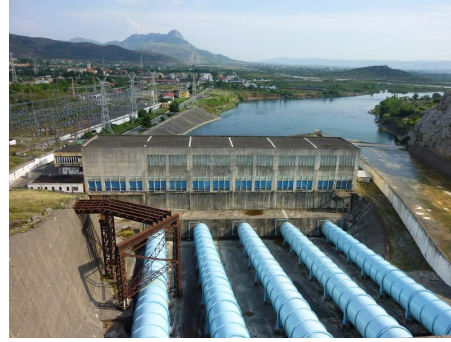
Figure 5: Pipelines (bottom), Power Generation Building (center), and Substation Facilities (upper left) (Vau i Dejes Hydropower Station)
