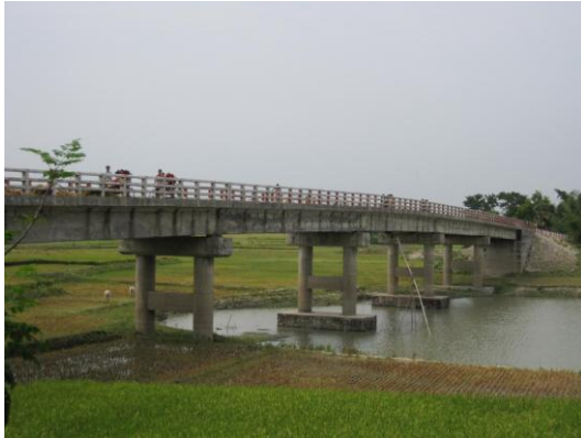
Photo 1. A Bridge Constructed under the Project (Jamalpur District)
