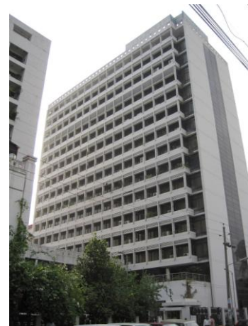
Photo 4: RDEC, built under the Project
