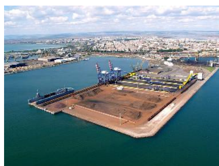
Terminal 2A at the Port of Bourgas
