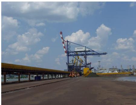
Figure 5: Berth No. 32 (in the far back is the ship unloader procured for the project)
