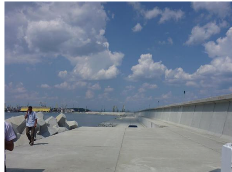
Figure 6: Breakwater Constructed by the Project
