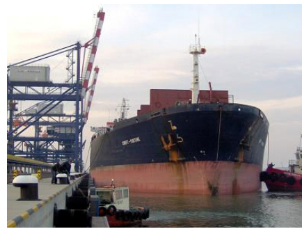
Figure 4: A vessel enters the Port of Bourgas. Vessels up to 120,000 tons may enter the port.
