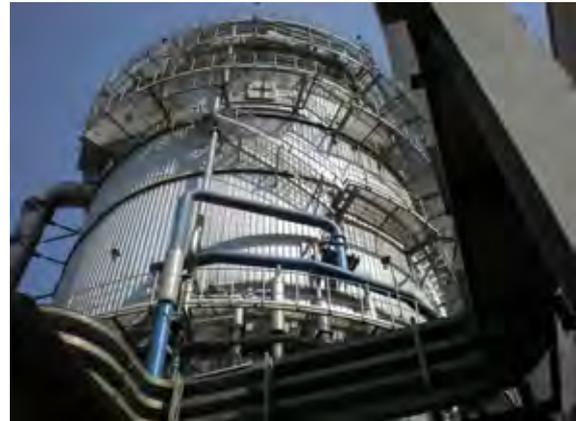
**Fig. 12: Smoke elimination/desulphurization equipment**
