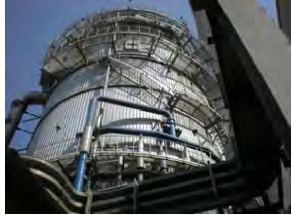
**Fig. 12: Smoke elimination/desulphurization equipment**
