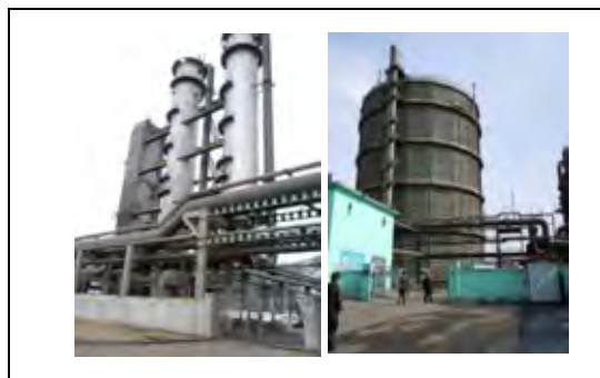
Beitai Iron & Steel Group (Left: coke oven environmental pollution control facilities, right: facilities for utilization of emission gas)
