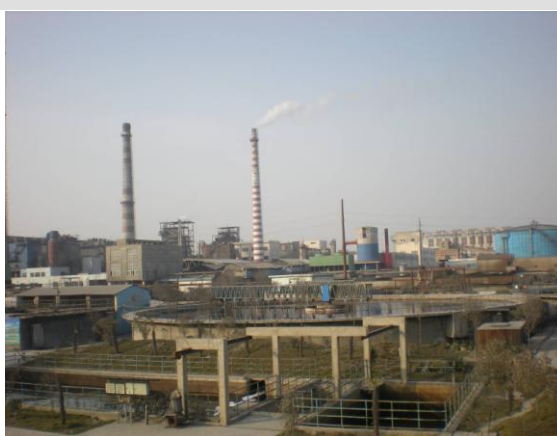
Louhe Pulp and Paper Making Factory
