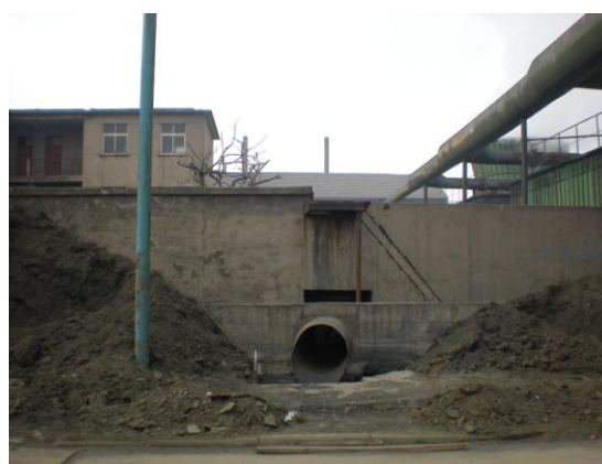
Fig.3 After Equipment Removal, Kaifeng Chemical Fertilizer Plant Waste Water Synthetic Treatment Project
