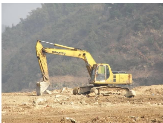
Fig. 8 Sub-project 4-2) Garbage Sanitary Filling Yard Construction Project in Changsha City: Equipment (a backhoe excavator)
