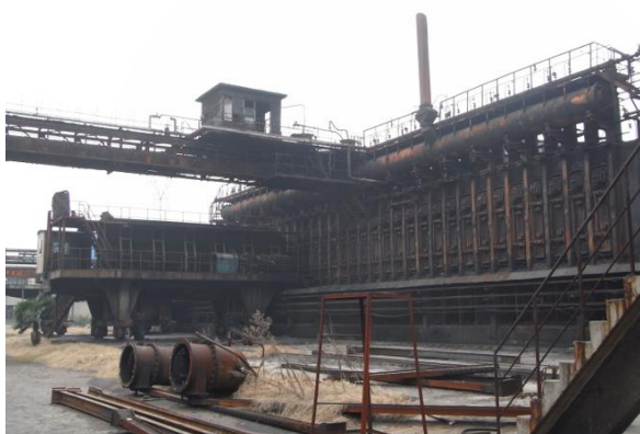
Fig. 6 Sub-project 3-2) Expansion Project of Gas Production Plant in Zhuzhou City: Added coke furnace (no longer in operation)
