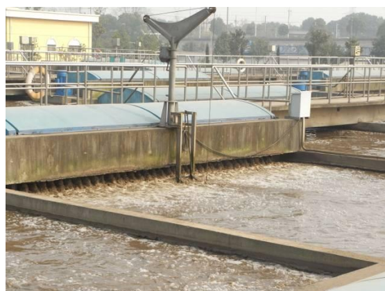
Fig. 3 Sub-project 1-8) Expansion Project of Changsha No.1 Sewage Treatment Plant: oxidation ditch process-based treatment facility
