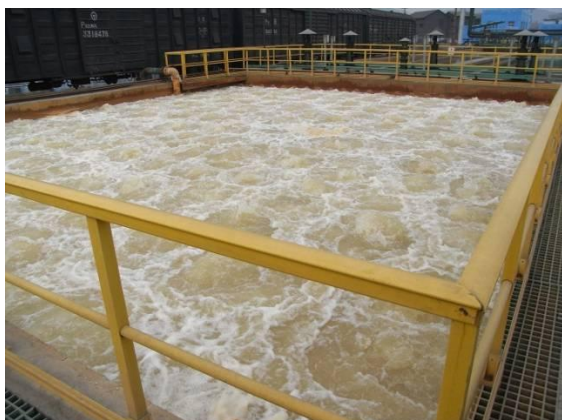
Fig. 4 Sub-project 2-2) Wastewater Treatment Project for Zhuzhou Chemical Factory: Compressed air is injected for sulfuric acid washing.
