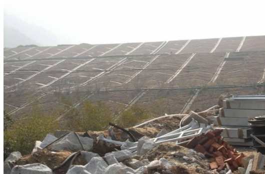
Fig. 9 Sub-project 4-2) Garbage Sanitary Filling Yard Construction Project in Changsha City: Filling yard side ditch
