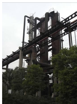
Fig. 7 Sub-project 3-2) Expansion Project of Gas Production Plant in Zhuzhou City: Added coal gas purification equipment (no longer in operation)
