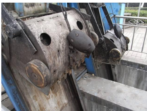
Fig. 2 Sub-project 1-6) Sewage Treatment Project in Xingsha Development Area of Changsha: wide-mesh screen
