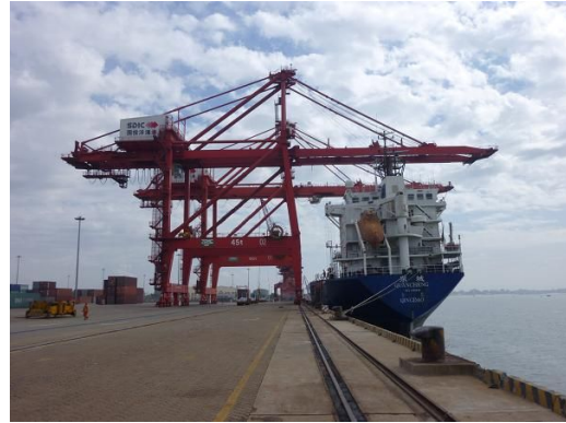
Container Berth in Yangpu Port
