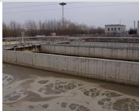
Mudanjiang Sewage Treatment Plant
