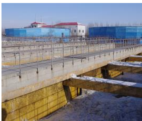
Fig. 2 1-3. Daqing Wastewater Treatment Plant
