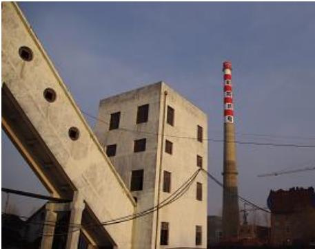
Fig. 5 Heat Supply Equipment in Jidong
