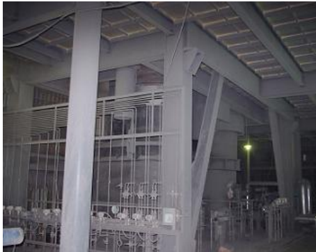
Fig. 4 3-2 Heat Supply Equipment in Yichun
