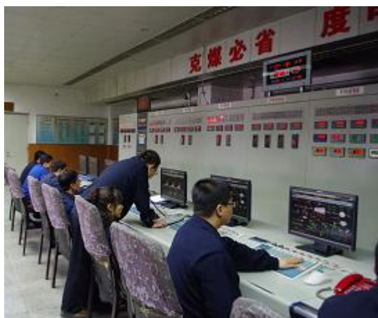
Fig. 6 3-2. Central Control Office of Mishan Heat Supply
