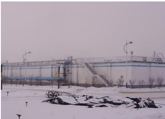
Fig.2 Sewage treatment plant in Songyuan City
