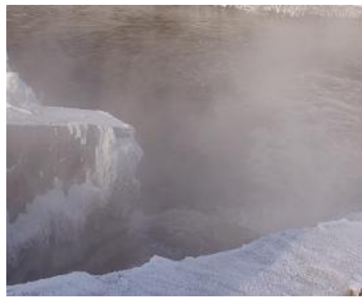
Fig. 7 Outlet of a sewage treatment plant
