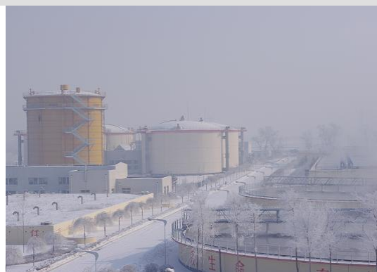
Sewage Treatment Plant in Jilin City
