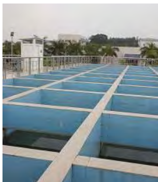
Nanning Sanjin Water Plant Flocculation Pond
