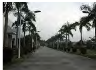
Sanjin Water Plant with green plants
