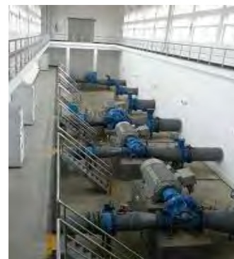
Guilin Chengbei Water Plant Pumps for transmission
