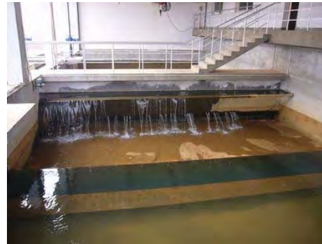
Jian (Wuyueguan Water Plant) Filter Basin
