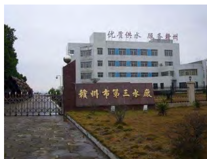
Ganzhou No.3 Water Plant
