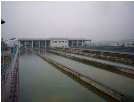
Nankang (No.2 Water Plant) Sedimentation Basin
