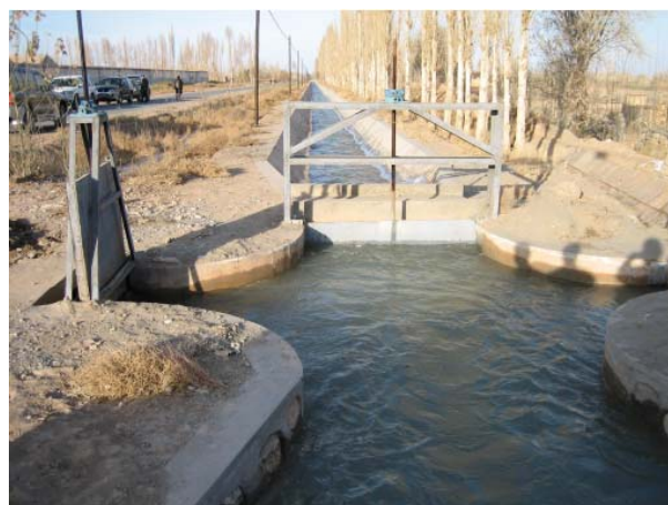
Completed canal with concrete lining
