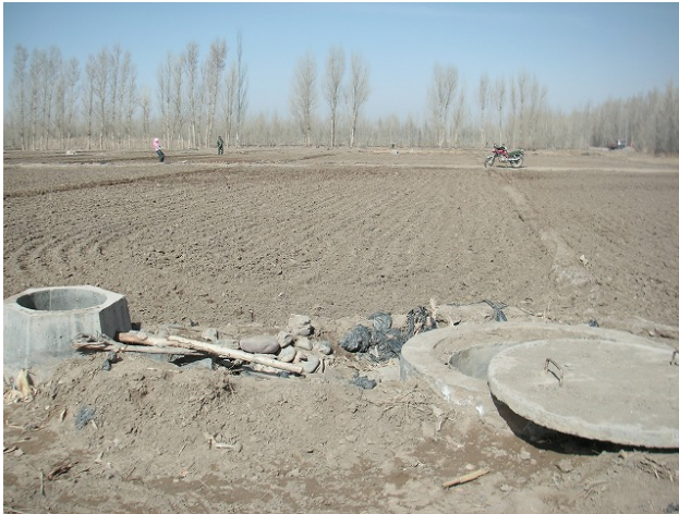
A one-mu farm is irrigated by a set of underground pipe irrigation facility whose concrete holes containing an outlet (left) and control valves (right) are installed on the ground. Farmers are doing land preparation for coming planting season.
