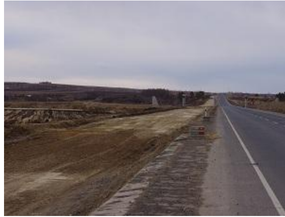
Fig. 3 Construction of Widening the Second-class Road
