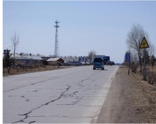
Fig. 14 Cracks on Road Surface
