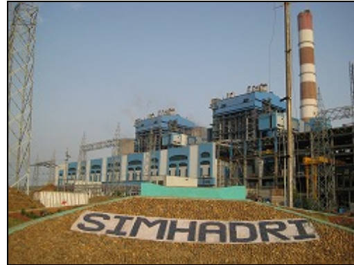
Simhadri Thermal Power Plant
