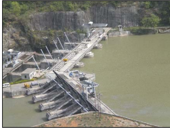
Photo: Water Intake Dam
