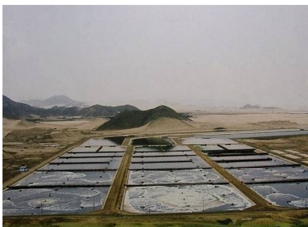
San Bartolo Sewage Treatment Plant
