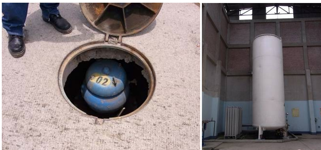
Gas exhaust port at the transmission line Oxygen tank for the transmission line
