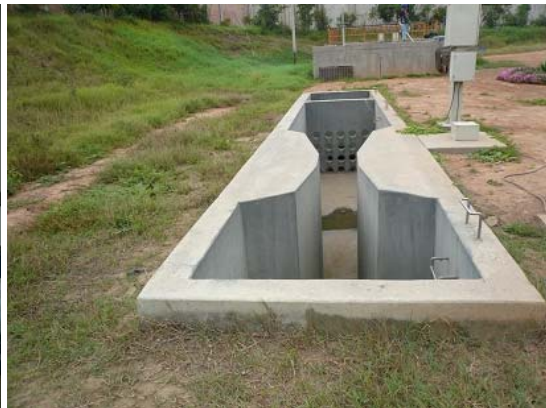
(Right) Receptor from the Transmission Line (not in use due to change in plan)
