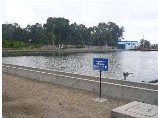
San Juan STP : Pre-Treatment Plant (left), Stabilization Pond (right)
