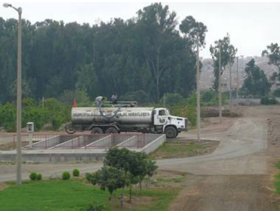
Water Truck receiving Water at San Juan STP
