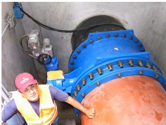
Connection between an existing Sewer and the transmission line
