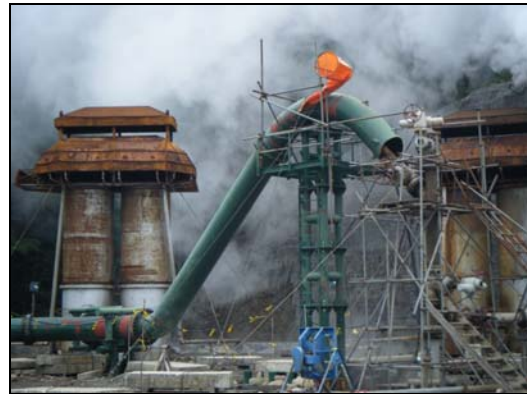
Photo 1: Production well under development
