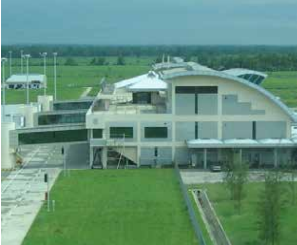
Passenger Terminal Built by the Project ( New Bacolod Airport )
