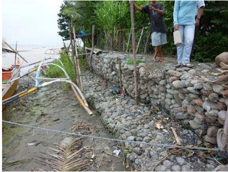
P-7. Buayan River Mouth gabion revetment
