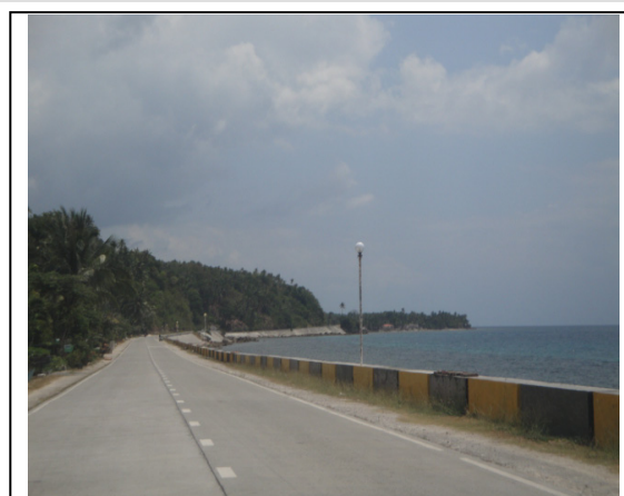
Project Road (Bohol Circumferential Road)
