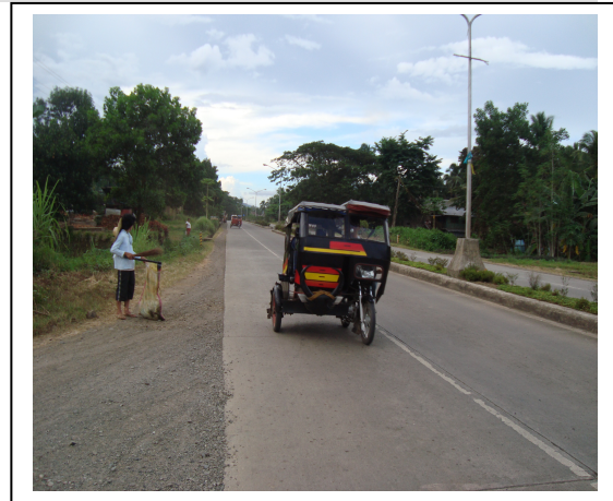
Road expanded to four lanes
