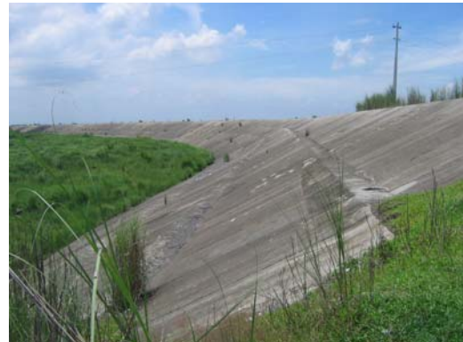
Southwest Mega Dike renovated by the project
