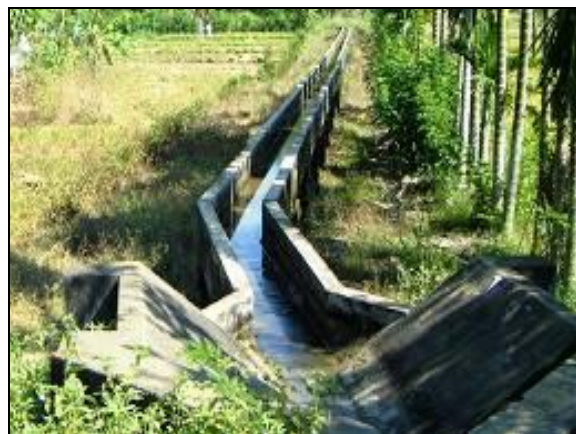
Rehabilitated D-F Canal of Irrigation Scheme
